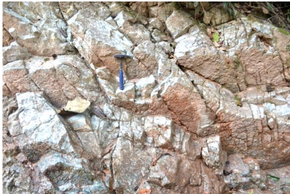
Figure 12: Joints cut the granite body in the study area resulting roughly angular fragments (“brecciation”)
