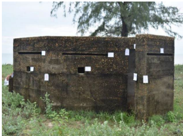
Figure 9: Pillbox in Kg. Ger, Bachok, Bachok, Kelantan
