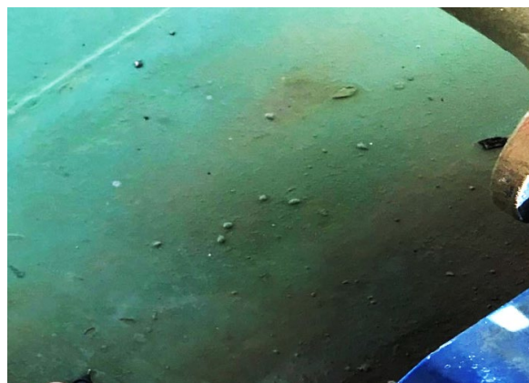
Figure 5: Blister rash on coating of RV-Discovery.
