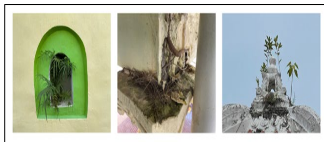
Figure 7: Ferns and Ficus species growing and thriving on the ventilation openings, beams, and roof crown of Serkam Pantai Mosque, Jasin, Melaka.
