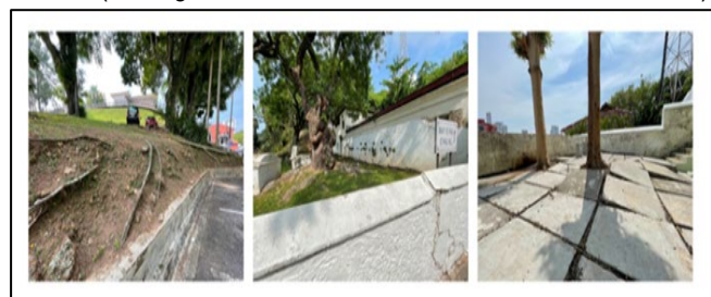
Figure 6: Exposed creeping roots can be seen damaging the nearby structure at the Old State Legislative Assembly Building, Melaka.
