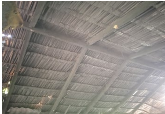
Figure 7: Palm thatch roofing in the existing langko at Pusa, Betong
