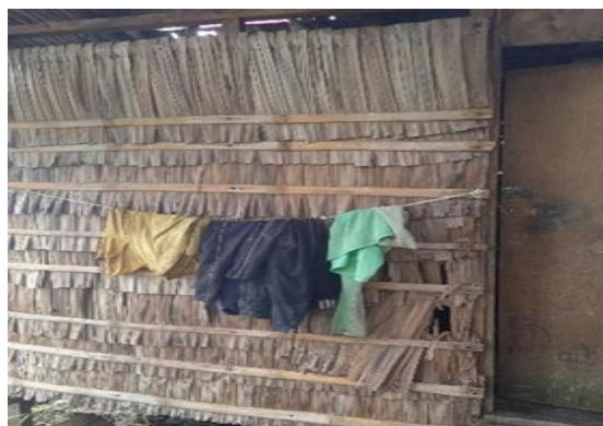
Figure 4: Small enclosed space at one side of the langko for storage
