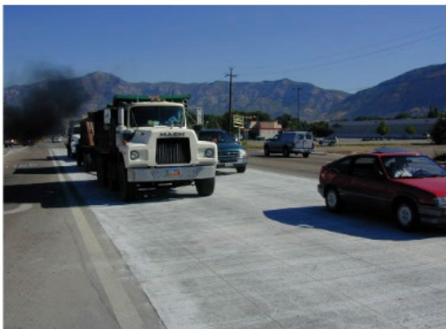
Figure 8: FRC bonded on asphalt used to construct streets and roads (Source: /view/dot/66993).
